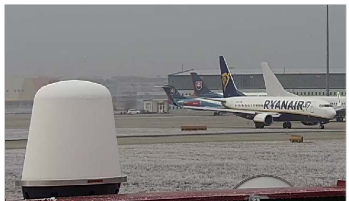
10 EHF Radar installation (white dome on the left)
