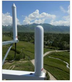
Secondary Surveillance Radar with the aim of helping secure air traffic safety in the area. ERA, as the primary contractor in co-operation with the local company Asiainfo, delivered its NEO multi sensor surveillance systems, a composite solution of multilateration and ADS-B technologies. The delivered system consists of nine ground stations with the expectation of an extension in the nearest future.
